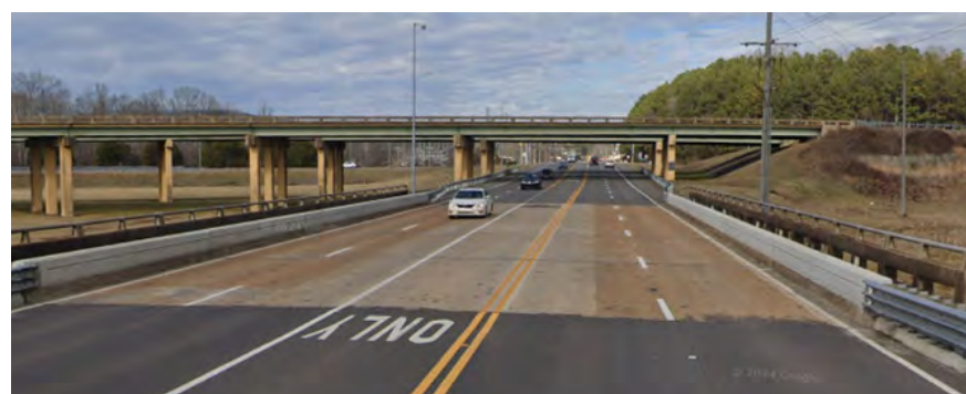
County HIN #5. South Broad Street underpass
