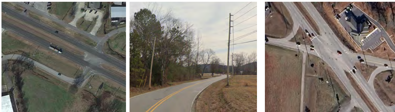
Unsignalized intersection at Little Cove Road; unlit double bend on County Highway 28; lack of crossing facilities at the Old Highway 431 intersection with US Hwy 431.
